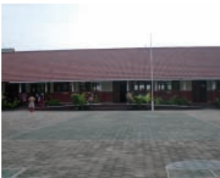
Giwangan State Elementary School after recovery in 2010
