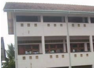
Relocated and newly built three-storey building
