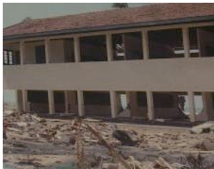
School damaged after it was hit by the tsunami
