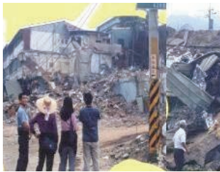
Piles of debris near Tong-Lin Elementary School
