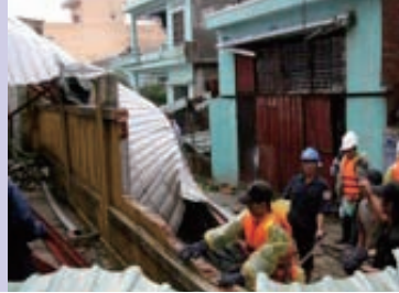
Cleaning and rebuilding after the typhoon
