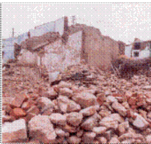
Vavaniya Kumar Shala School damaged in the earthquake
