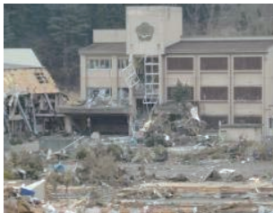
Damage at the Toni Elementary School
