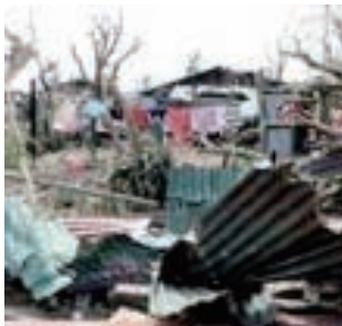
All the houses in Maconacon were damaged
