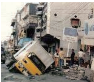
Several areas in Dagupan experienced serious liquefaction
