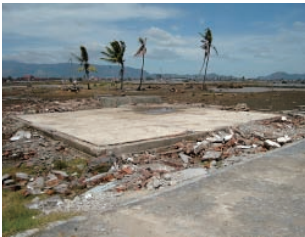
The devastated area of SDN 81 Tibang, Aceh
