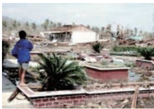
Maconacon Central School was totally destroyed
