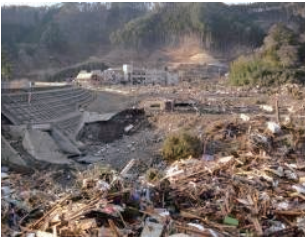
Damage at the Toni Elementary School
